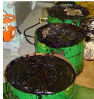
Sludge removed from purification system cleaning.
